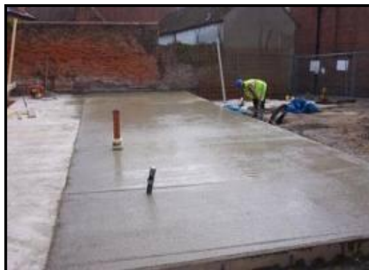
Concrete setting. This reaction is quite slow. It will take a couple of days for the concrete to harden
